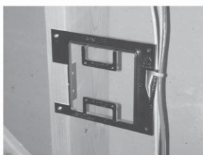
Figures 2 and 3: Photos of a Typical ZAC-60 Rough-in Bracket Installation
